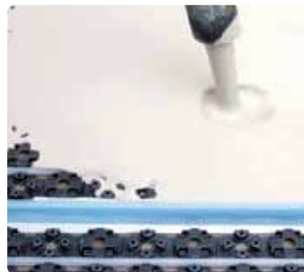
Levelling compound can spread easily
